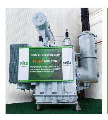
"Through winding structure and main insulation optimization, exit turret simulation improvement, cooling system verification and other research, 750kV natural ester transformer passed the rigorous third party witness tests, it reflects CHINT's capabilities in designing complex insulation systems and manufacturing ultra-high voltage transformers, it also verified the feasibility of using natural ester transformer up to a 750kV voltage level."
