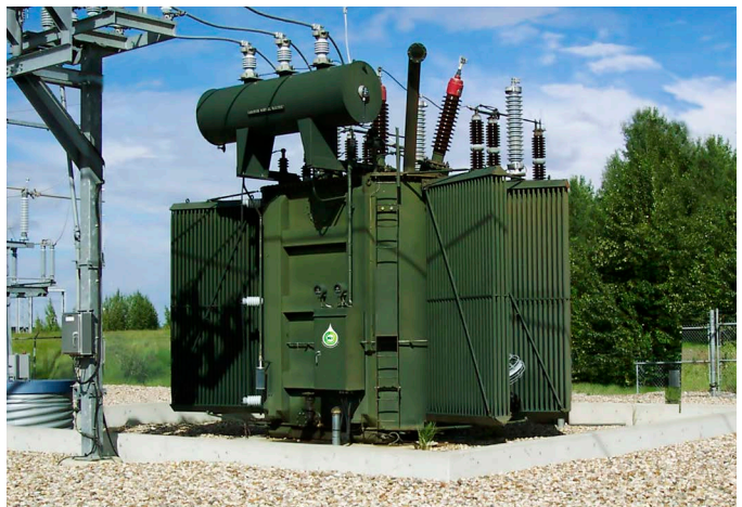
FR3 fluid has been used in distribution and power transformers through 420kV.
