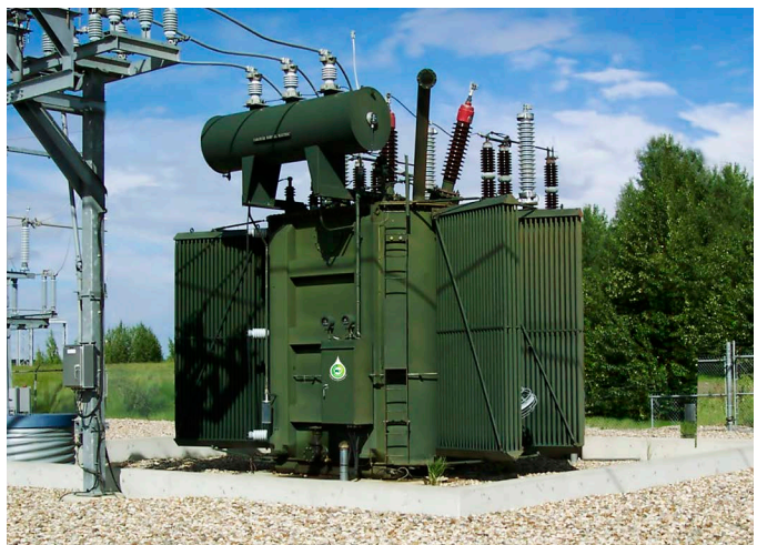
FR3 fluid has been used in distribution and power transformers through 420kV.
