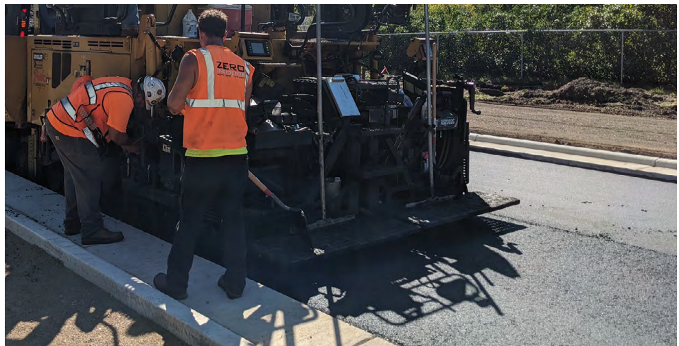
Wright County paving crew laying down asphalt with Cargill's Anova® Warm Mix Additive.
