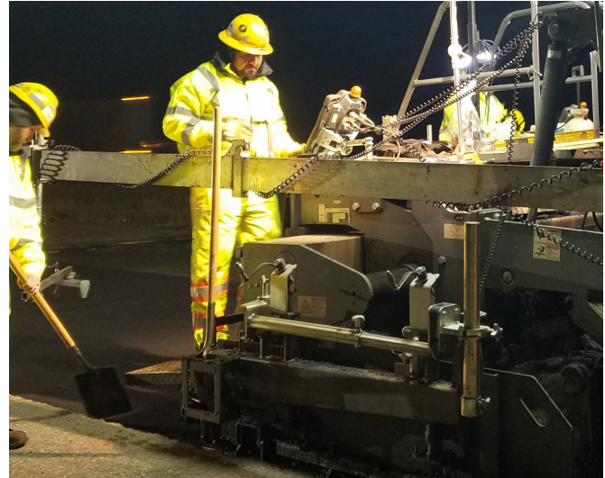
Paving crews laying down Cargill's Anova® Rejuvenator.
