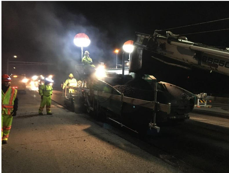
Figure 2 – Night Construction of 2018 Cargill Partnership test sections on I-94 at MnROAD
