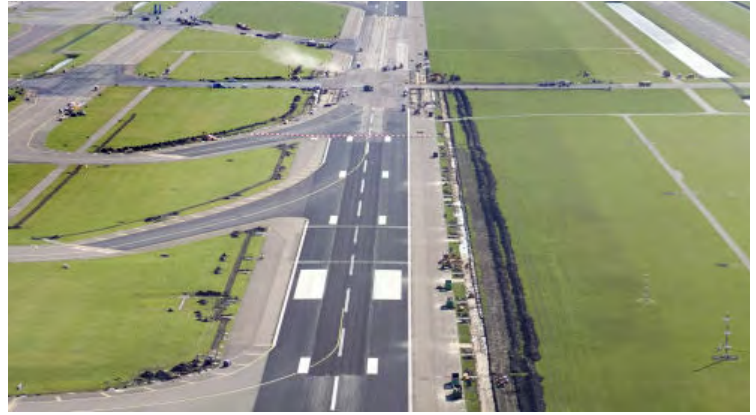
Overview of the paving project at the Polderbaan, with Cargill's Anova® Rejuvenator. © 2021 Heijmans
