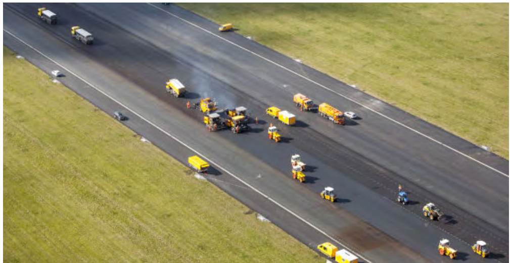
Heijmans paving the Polderbaan with Cargill's Anova® Rejuvenator. © 2021 Heijmans
